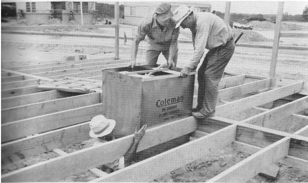
An oil burning floor furnace is put into each house before the flooring is laid.
