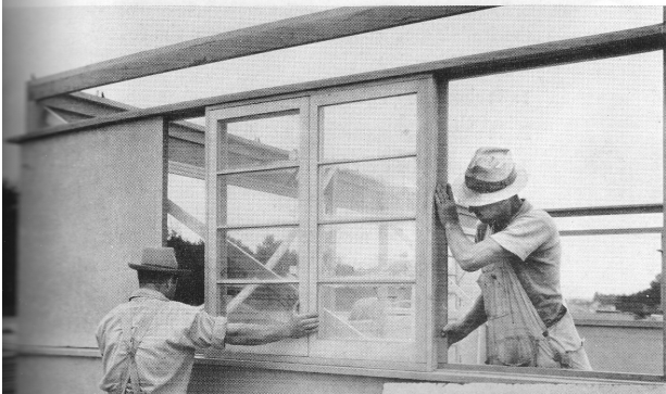
A wood casement window, complete with frame, is slipped into place.
