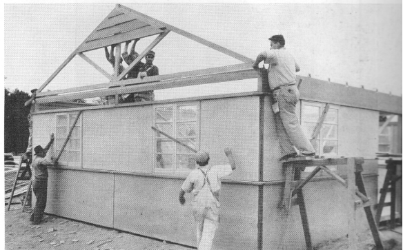
An end roof truss, equipped with ventilating louvres, is fitted into position.
