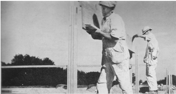
Tops of the columns are bound together with wood girders.
